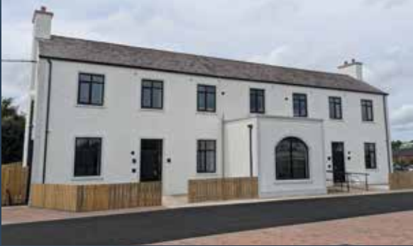
The Fever Hospital, the only standing remains of the Ballycastle Workhouse.
