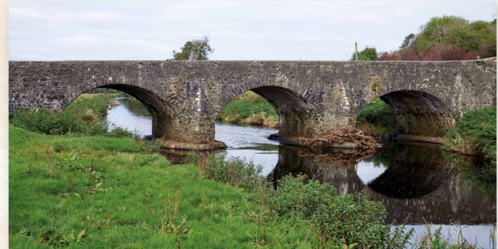
Seneril Bridge over the River Bush on a calm autumn day. The 'washed up debris' on one of the central piers shows the reason the arches are so high.
