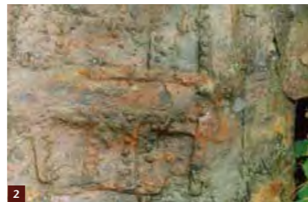
1 A typical C18th salt works. 2 The repaired bottom of a salt pan.
