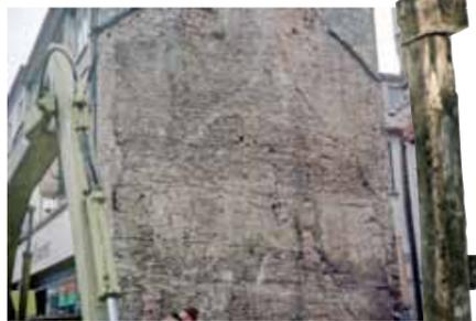
▲ Demolition in Church Street in 1985 revealed the 17th-century timber structure buried in more recent brickwork. Image courtesy of NIEA
