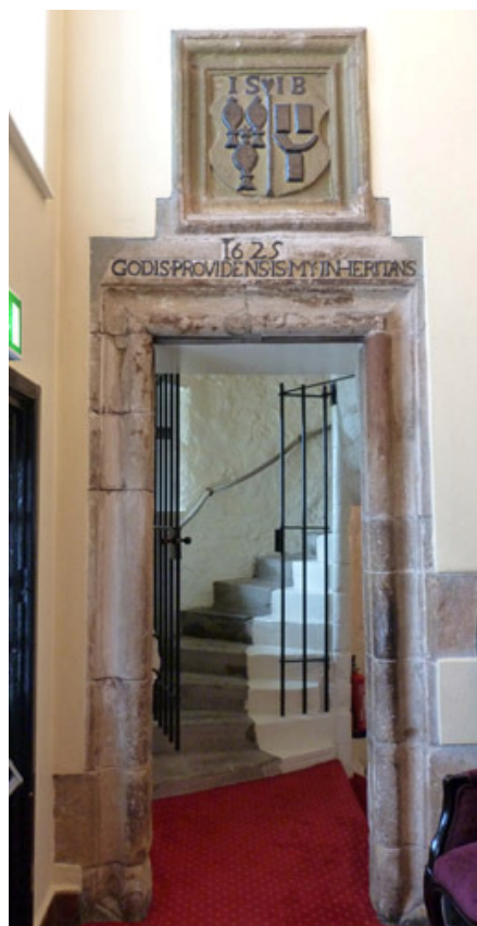
Interior doorway showing spiral staircase.
