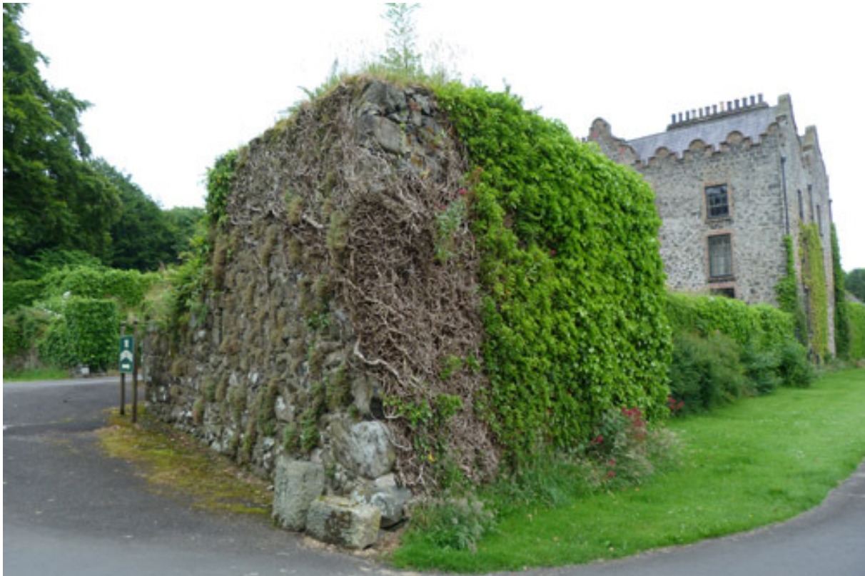
Flanker tower and bawn wall
