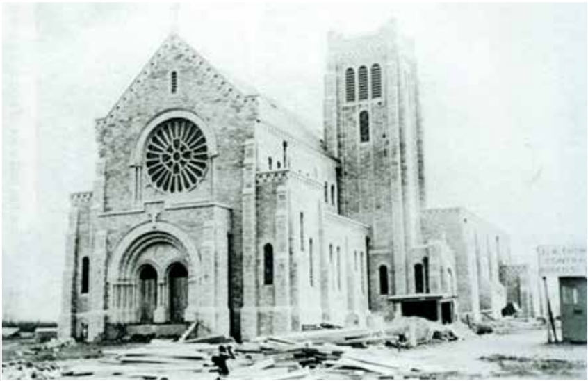
St Malachy's Church, Coleraine, during construction.
